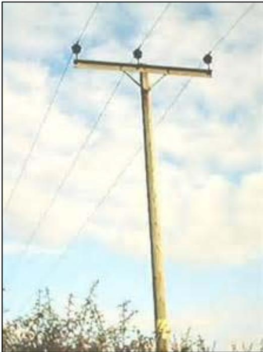
Figure 2 11 kV distribution line
