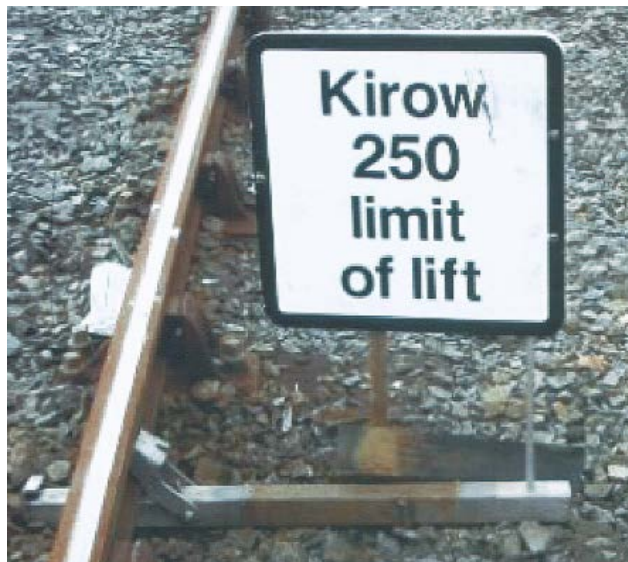
Sign indicating end of permissible lifting area or end prior to exclusion zone at underbridge
