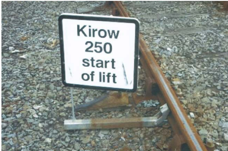
Sign indicating start of permissible lifting area or restart after exclusion zone at underbridge.
